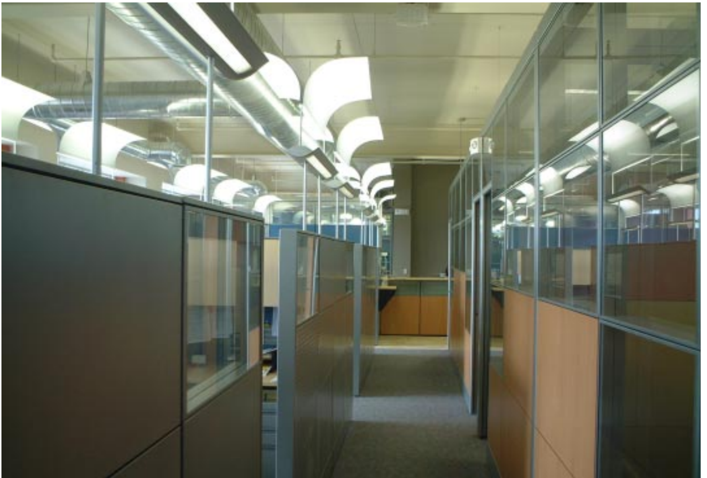
Coldwell Banker, Canada System MXi, System MXV2 & MXV2 System Wall - 300 Workstations
